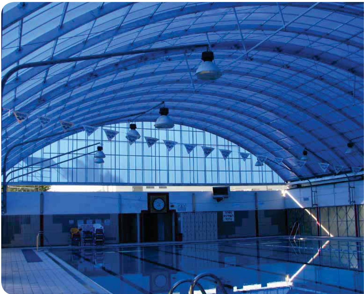
Roofing, Swimming Pool, Polyshade Blue
