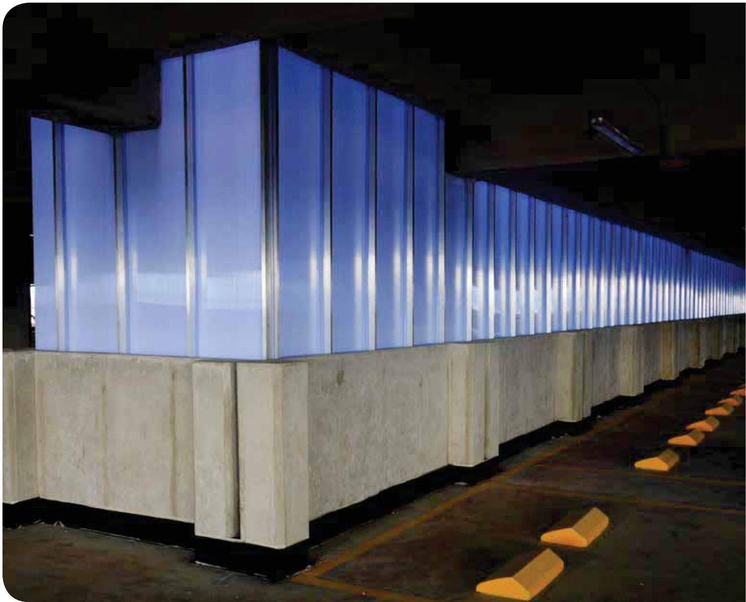
Cladding, Parking Lot
