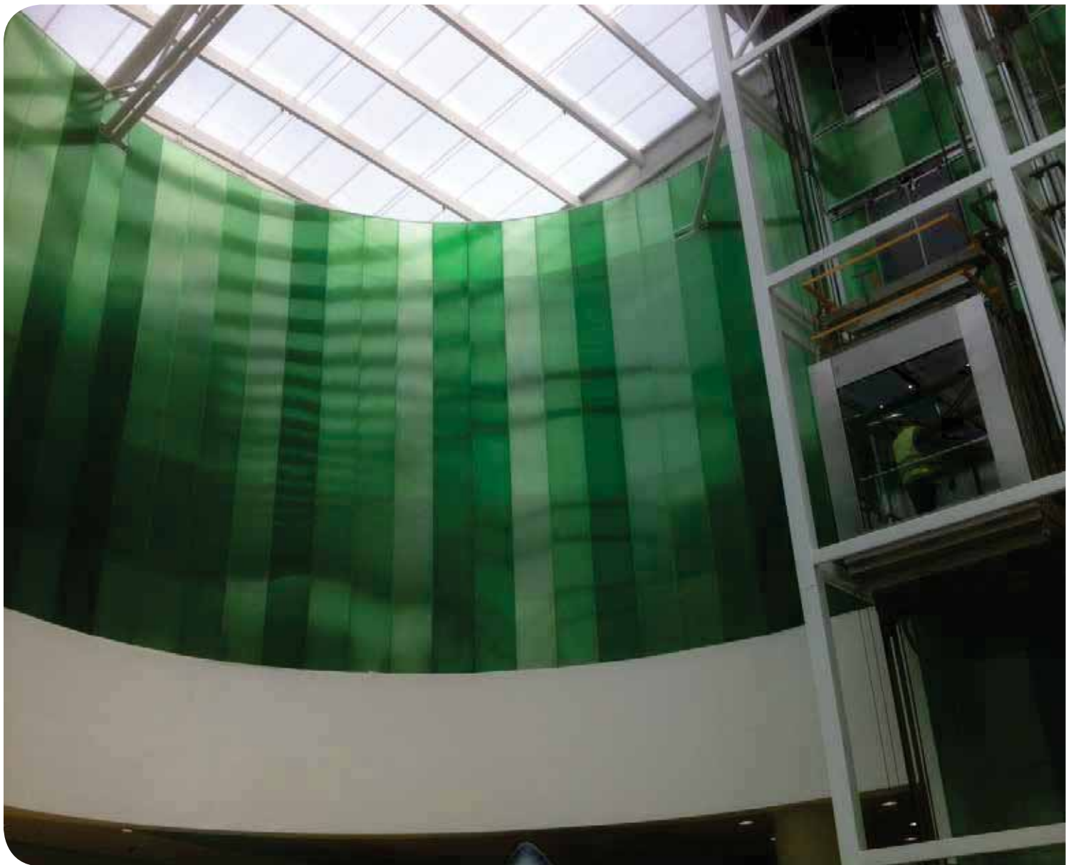
Cladding, Commercial Center Interior
