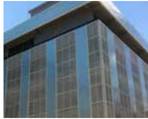
Roofing and windows
