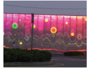
Lighting, Illumination and signage
