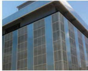
Roofing and windows
